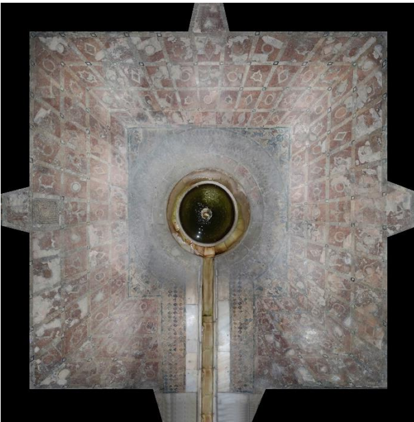
Figure 7: Top view of the floor mapped with multiple ortho-rectificated shots. The Pavillion of Charles V.
